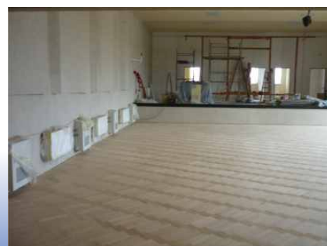
Remont sali GOK
